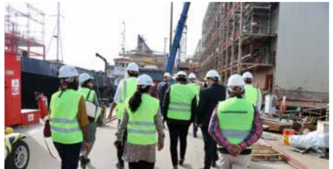
Members of Parliament on a site visit of Kapowership, a Turkish company that builds and operates floating power plants on ships.
